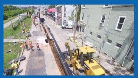
Exelon is focused on actions to reduce operational GHG emissions, such as replacing older cast iron and bare steel gas pipes to reduce fugitive methane emissions from natural gas distribution.
