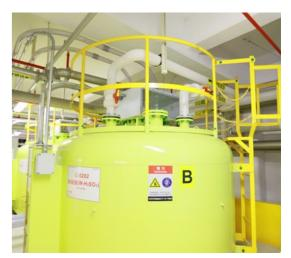
Waste Sulfuric Acid Recycling System
