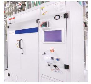
High-Efficiency Air Treatment Equipment (Local Scrubber) Dual Zeolite Rotor Concentrators
