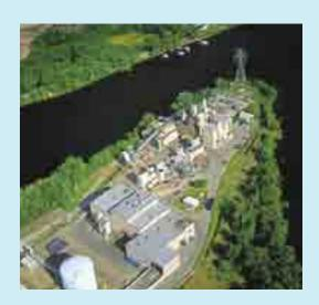
We have three power plants—the Red Wing and Wilmarth Generating Stations in Minnesota and the French Island Generating Station in Wisconsin—that produce about 53 MW of electricity from fuel derived from municipal solid waste or garbage, called refuse-derived fuel (RDF).
