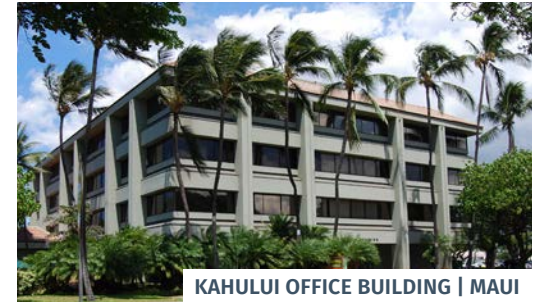
KAHULUI OFFICE BUILDING | MAUI
