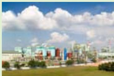
The installation of a methanol recovery plant at the Riau pulp production mill is APRIL's first Clean Development Mechanism (CDM) project. The project entails the collection of non-condensable gases (NCG) from the black liquor evaporators, traditionally flared, and condensing and concentrating the methanol constituent from other inert gases. The concentrated methanol
