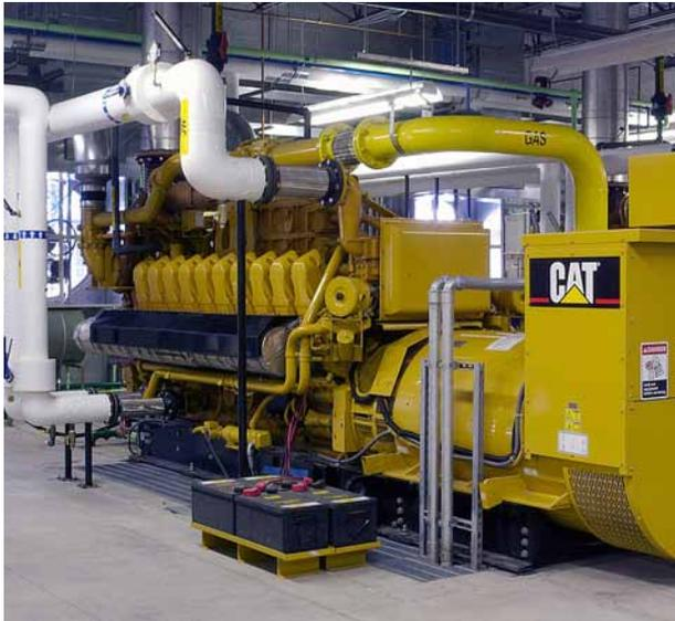
and through the capture and combustion of methane gas produced in our landfills. Five of our landfills are equipped with Landfill Gas-to-Energy facilities. These energy facilities are designed to produce roughly 25 megawatts of clean energy.
