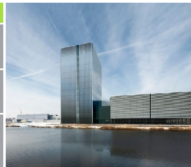
AM4 Amsterdam IBX® Data Center
