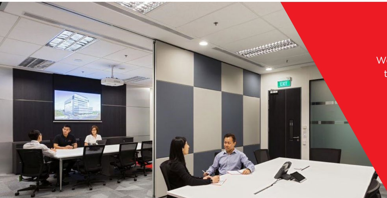
SG3 Singapore IBX® Data Center
