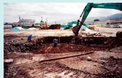
Photo 2 Soil cleanup at former Epson Logistics Head Office site
