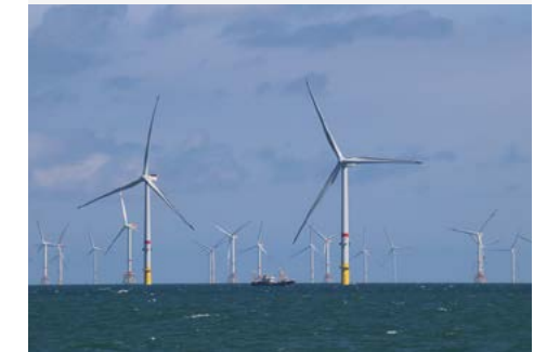
© Norther wind farm off the coast of Belgium and the Netherlands provides renewable energy for our operations in both countries.
