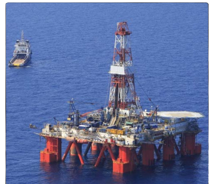
Hakuryu V drilling rig, Vietnam
