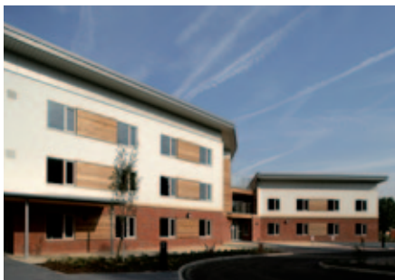
Care home at Bromford Lane, Birmingham built using Space4 technology
