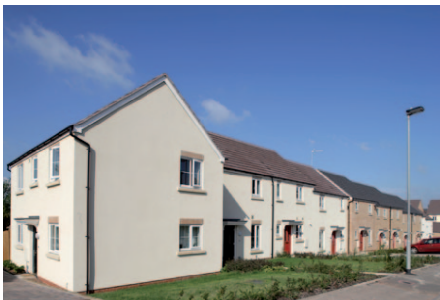
Persimmon built 82 new homes to high environmental standards and with low carbon emissions, achieving Code Level 3 at Windsor Road, Redditch
