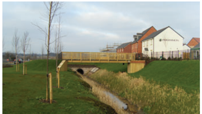
Above A typical SUD system constructed at our site in Llanwern, Newport
