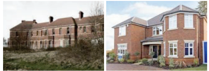
Above Redeveloping a former hospital at Hellingly, East Sussex
