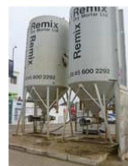
Figure 18 – Mix mortar silo on one of Persimmon Homes' sites on the south coast
