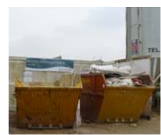
Fig16 – Waste segregation facilities on a site
