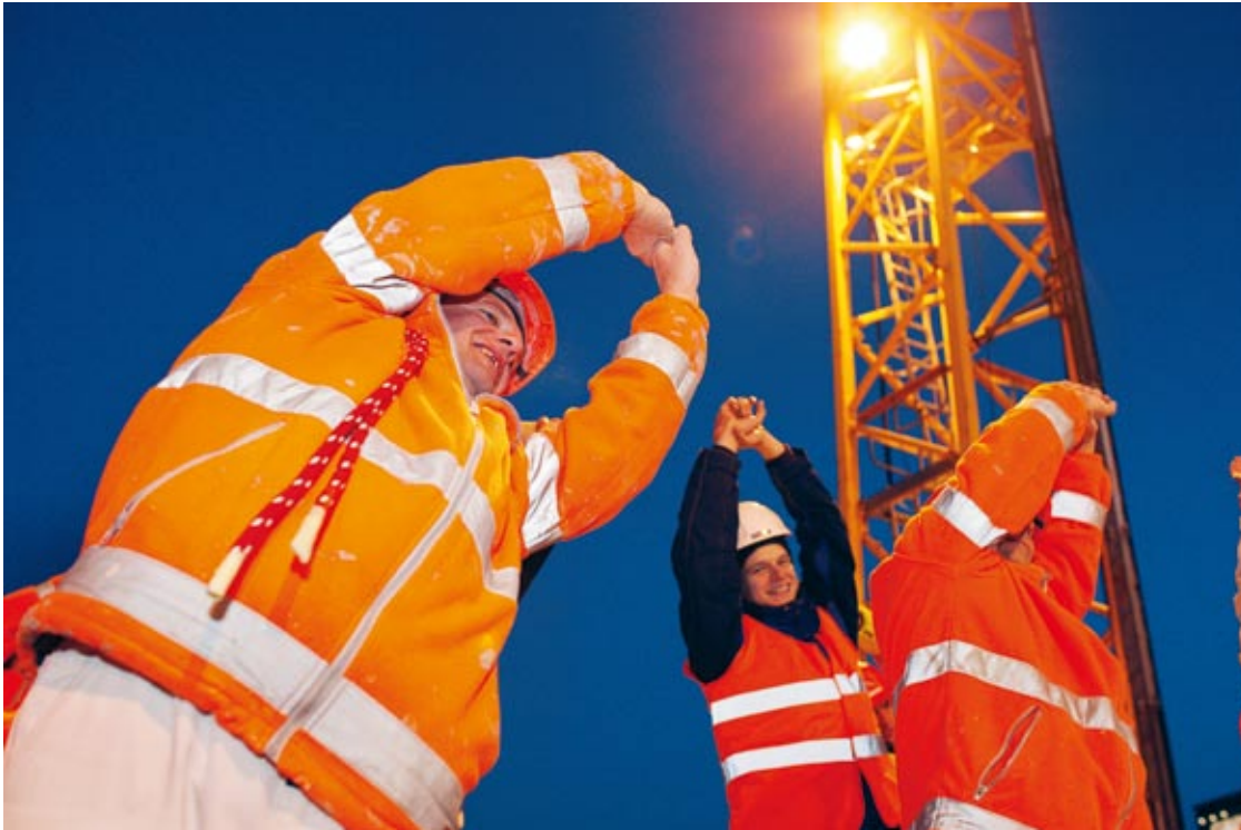
One health and safety initiative is group warm-up exercises, which take place at the beginning of the working day. In many projects, “stretch and flex” exercises have helped decrease back problems among employees.
