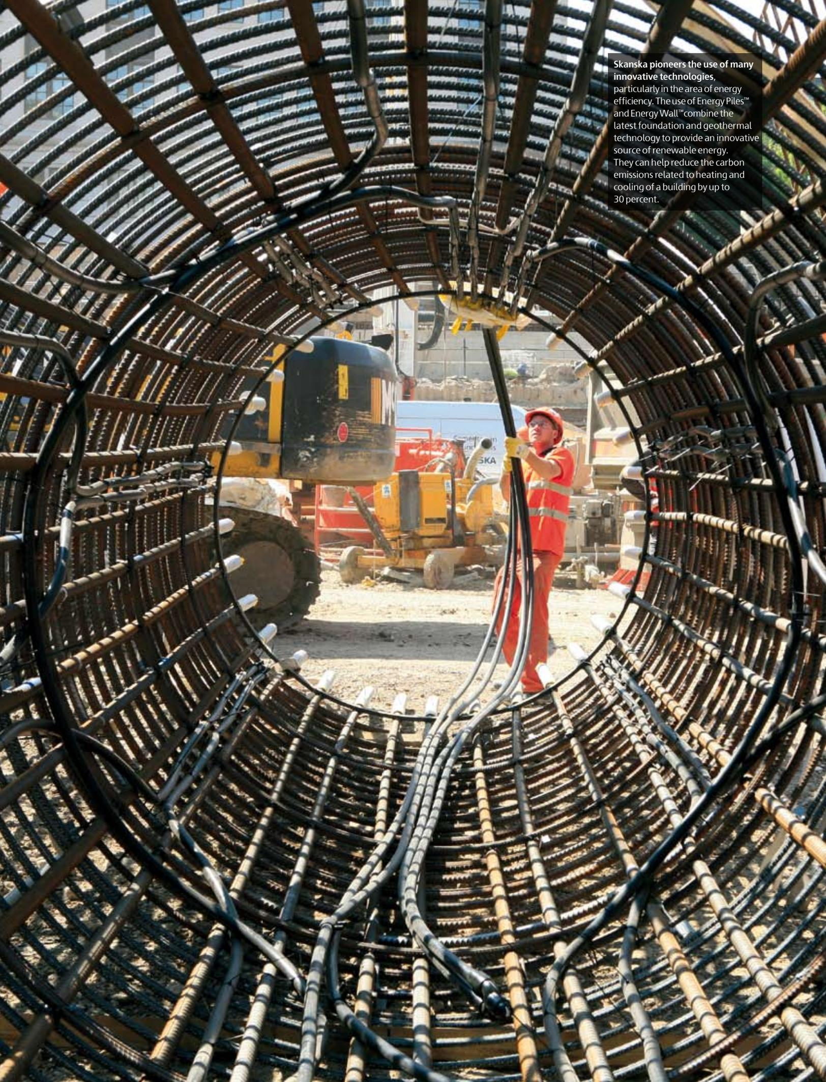
Skanska pioneers the use of many innovative technologies, particularly in the area of energy efficiency. The use of Energy Piles™ and Energy Wall™ combine the latest foundation and geothermal technology to provide an innovative source of renewable energy. They can help reduce the carbon emissions related to heating and cooling of a building by up to 30 percent.
