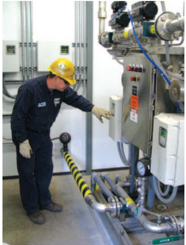
Assistant Control Operator Mark Sheets inspects the density set point on the Urea Concentrate Pump controls on the newly installed SNCR system at Centralia.
