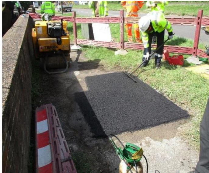
Figure 10 – Trial of the use of pelletized waste plastic in an asphalt mix
